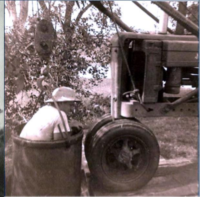
HORACE IN THE BUCKET EXCVATING HAND-DUG WELL, 1965
