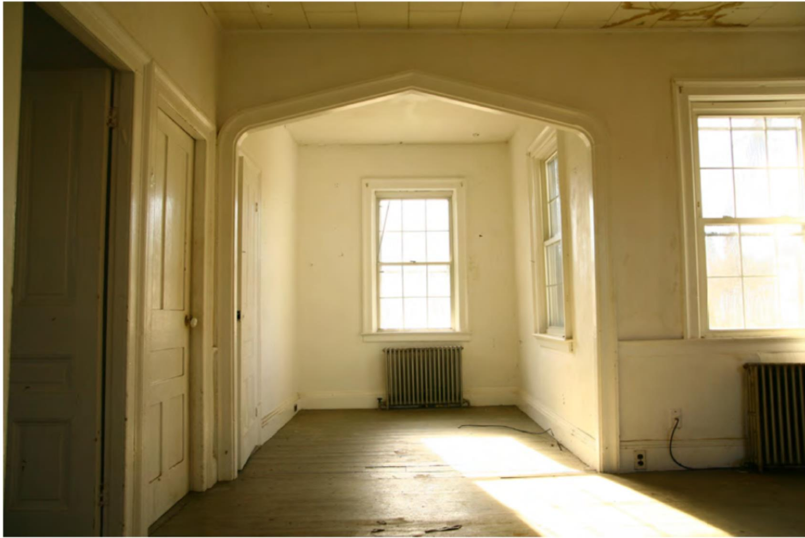
Fig. 24. The Gothic Revival arched opening between the kitchen and this alcove appears to be original to the construction of the house and shares architrave profiles found at the door and window openings on the first floor. The Greek Revival and Gothic Revival styles coexisted simultaneously, and occasionally builders employed elements and details interchangeably.
