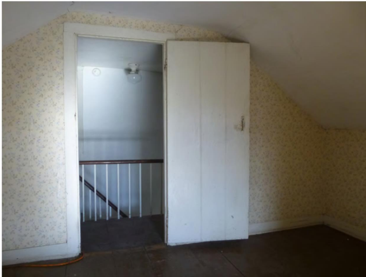
Fig. 25. Unlike the stylish treatment of the first floor rooms, the chambers have little in the form of decorative treatments, Doors throughout are board and batten with surface latches.
