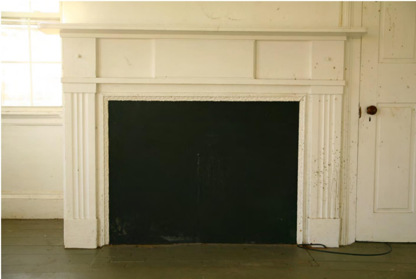
Fig. 19. South parlor, mantelpiece Compare this element to that illustrated in Asher Benjamin's, The Practice of Architecture, Plate 47 (Fig. 3). While the embellishments differ, the overall composition is very similar.
