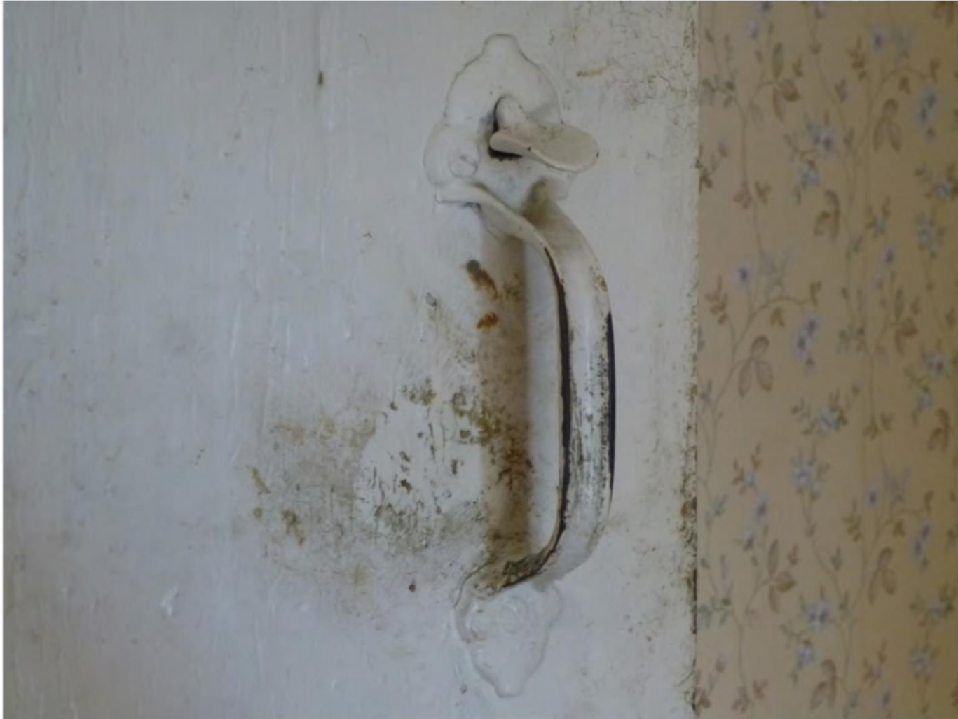
Fig. 26. Detail of a cast iron Blake latch found throughout the second floor level. The design for this latch was patented in 1840.
