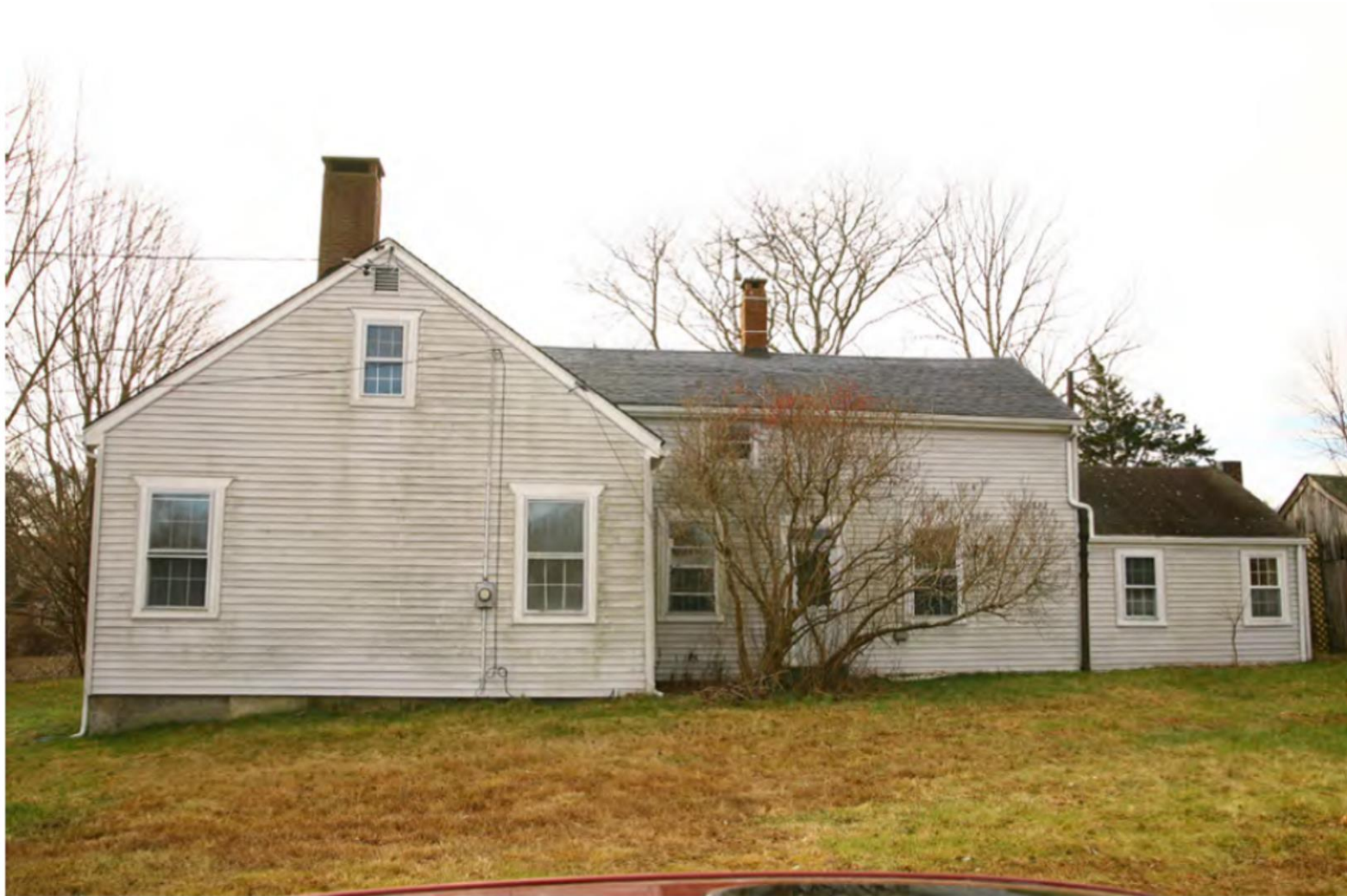
Fig. 7. Helfand house, north elevation showing ell and circa 1875 addition at west end. December 2014.
