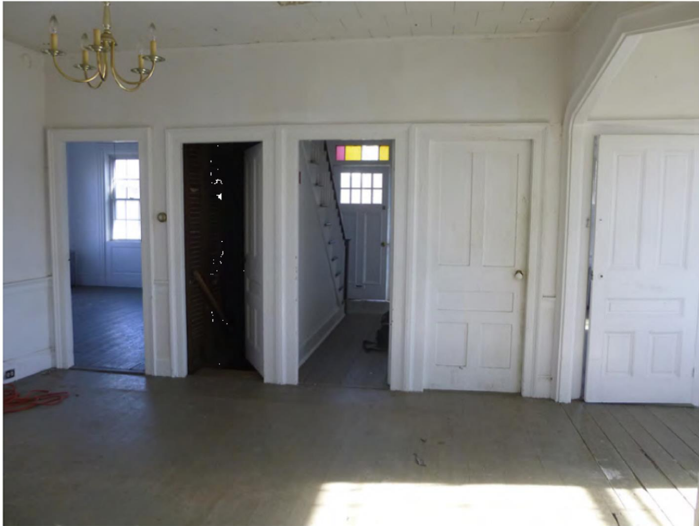
Fig. 23. Kitchen, east elevation showing the series of five doors. The door at the left of the image was added sometime in the last quarter of the nineteenth-century.
