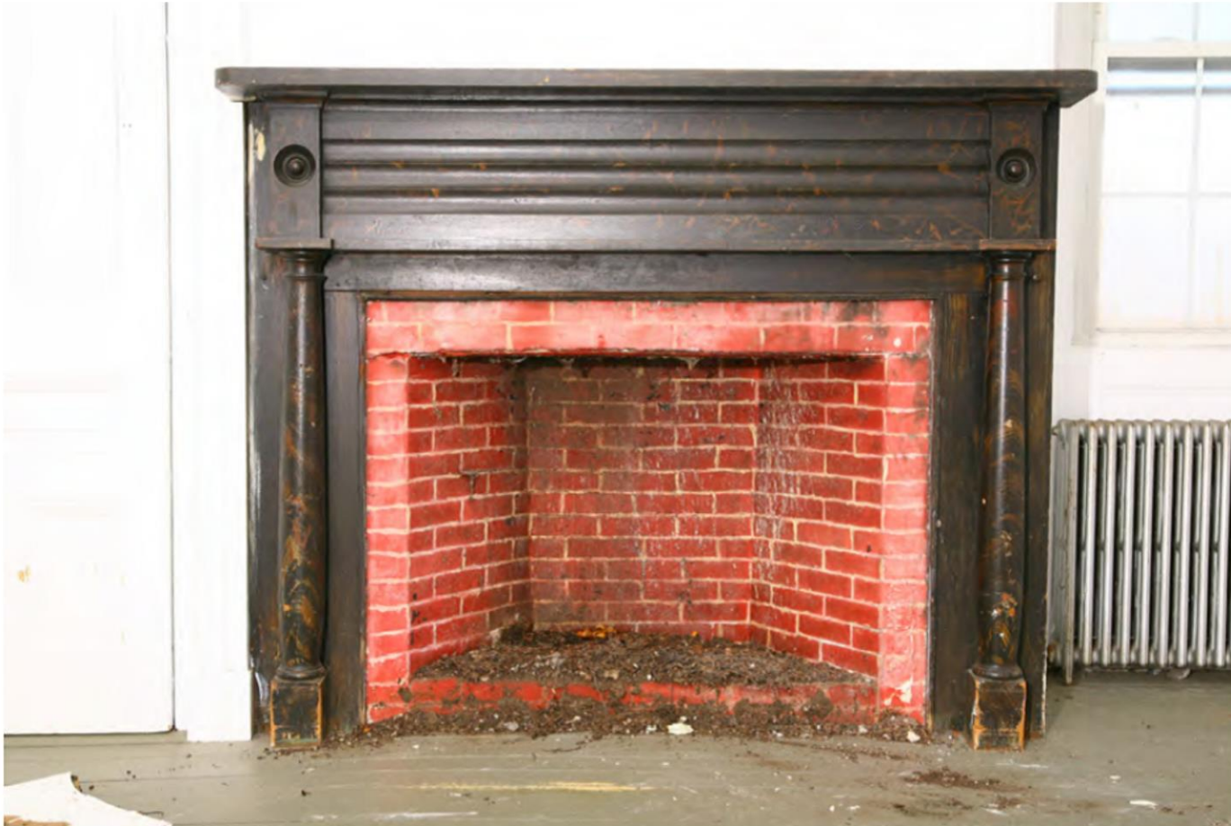
Fig. 16. North parlor, mantelpiece. The mantel is a fine representation of an early Greek Revival piece complete with its early faux marble paint finish. The firebox exhibits classic Rumford proportions. Mounts for a crane remain in the masonry of the west splay. Two courses of brick have been added across the opening of the hearth. It is interesting to see that the house employed fireplaces rather than cast iron stoves which were becoming widely available when the house was constructed.
