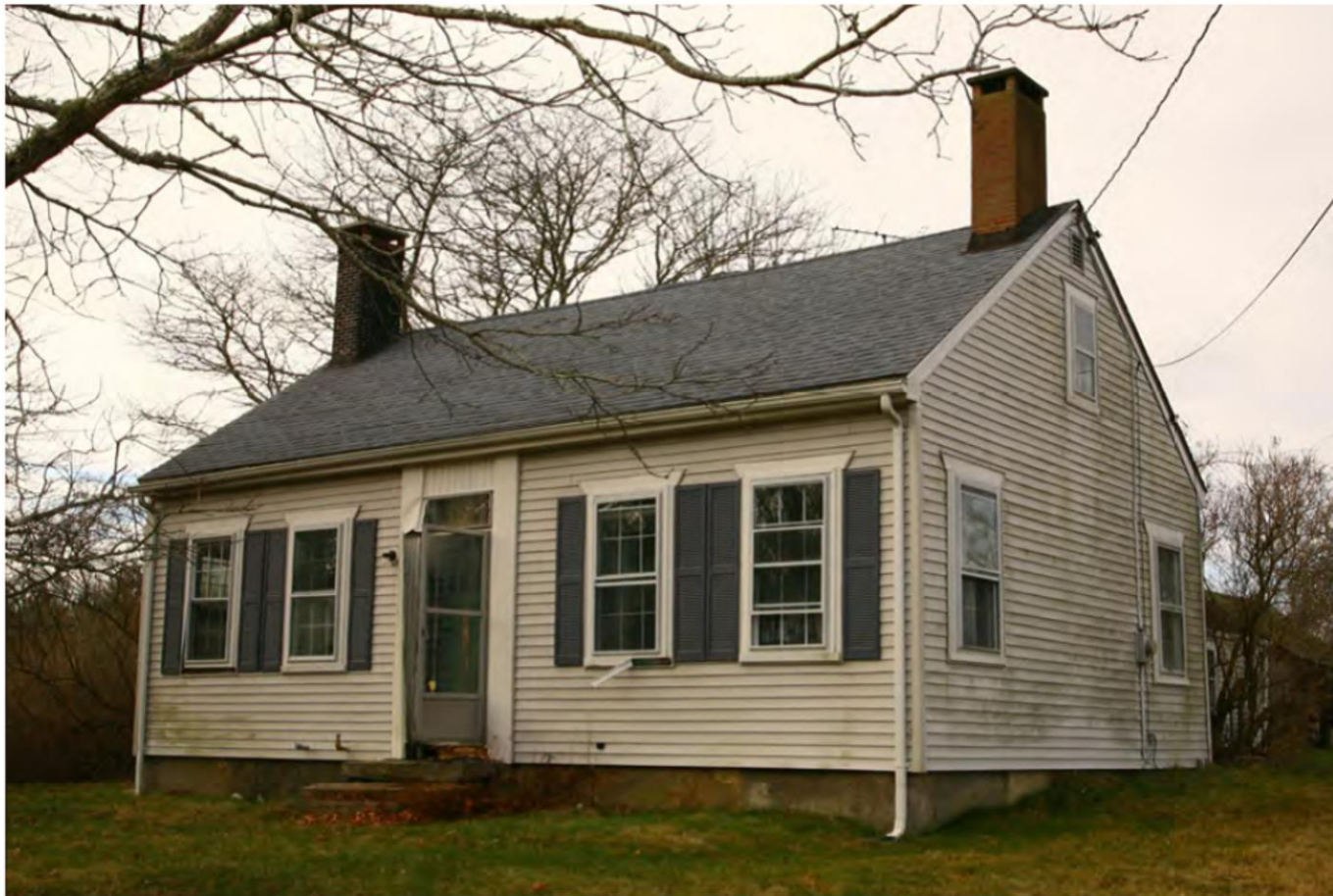
Fig. 6. Helfand house, north (gable) and east elevations. December 2014.
