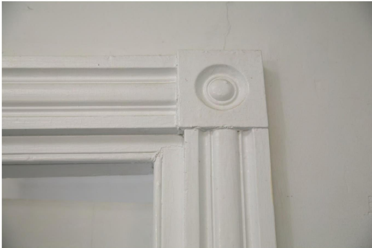
Fig. 13. North parlor, typical architrave found in the room. Note the corner block and compare to the windows shown in Benjamin's, The Practice of Architecture (Fig. 4)
