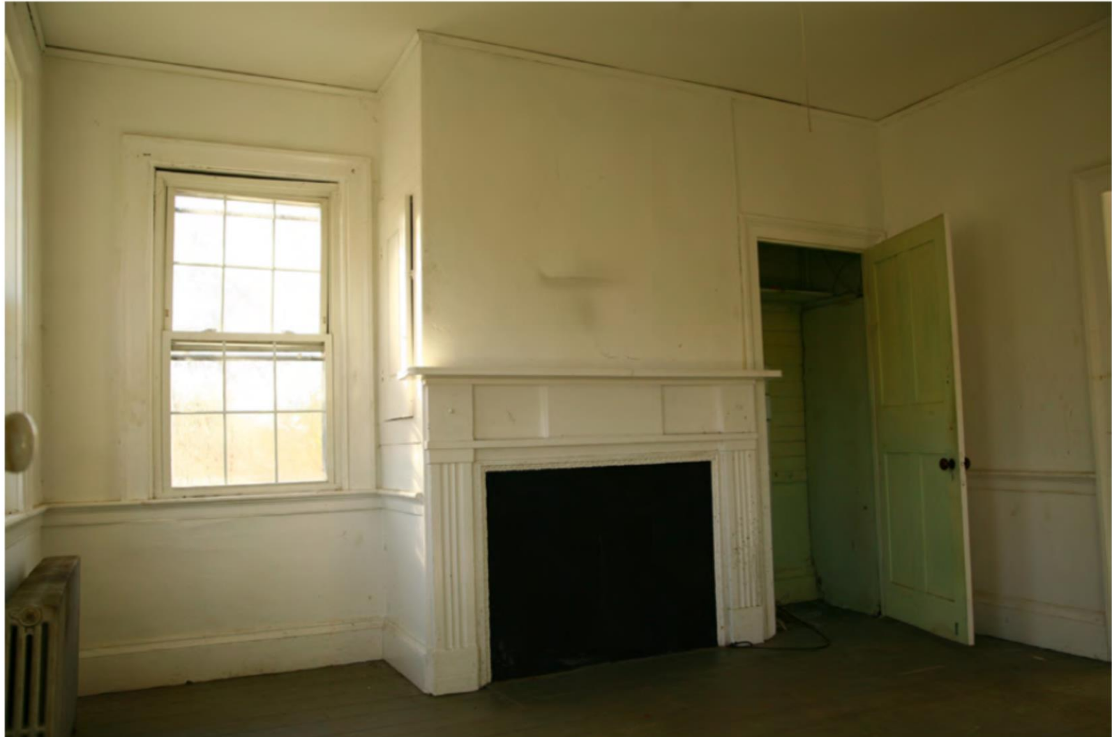
Fig. 18. South parlor, south elevation. Features to note include the original closet, built-in cabinet on the side of the chimney breast, mantelpiece, window architrave, surbase (or chair rail), and base (or base board).
