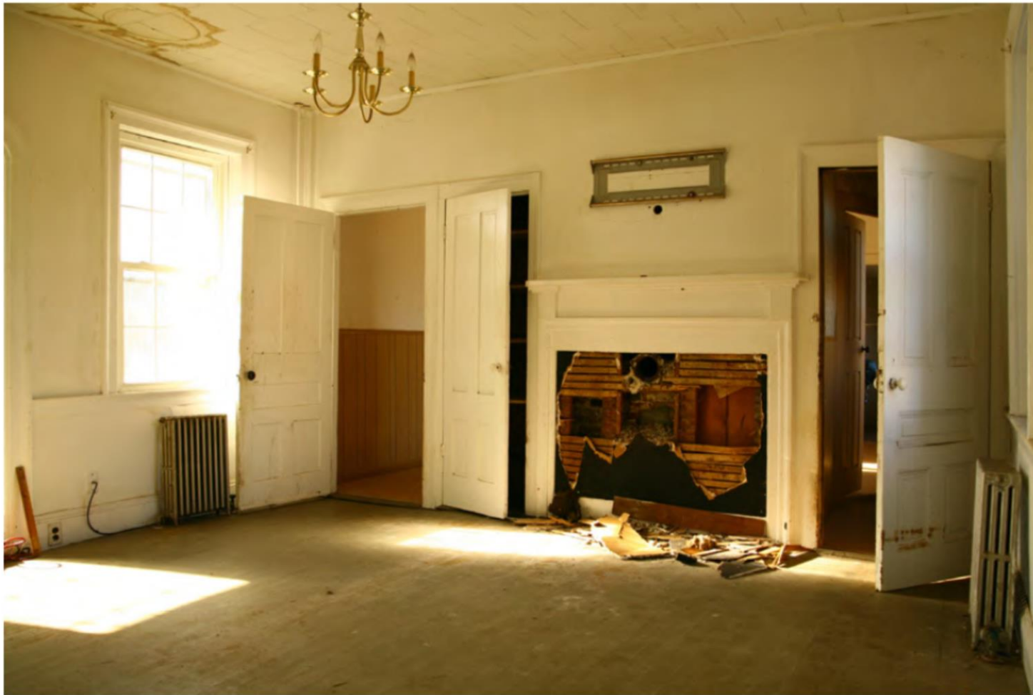
Fig. 22. Kitchen, west elevation. Unlike the parlors which retained fireplaces, the kitchen originally utilized a cook stove which would have plugged into a stove chimney behind the mantel. While there was no functional need for it, mantels continued to be used as architectural elements to frame stoves long after fireplaces disappeared.
