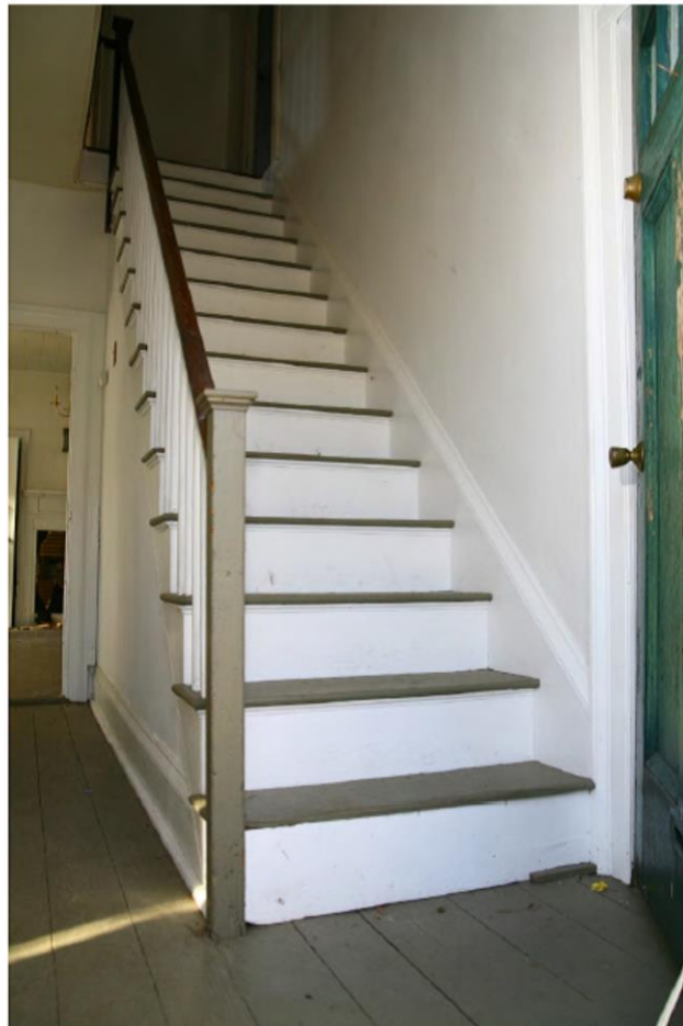
Fig. 11. The stair is original to the construction of the house; however, it has had some repairs done to it. All of the repairs remain faithful to the original design and have not detracted from the integrity of the piece.
