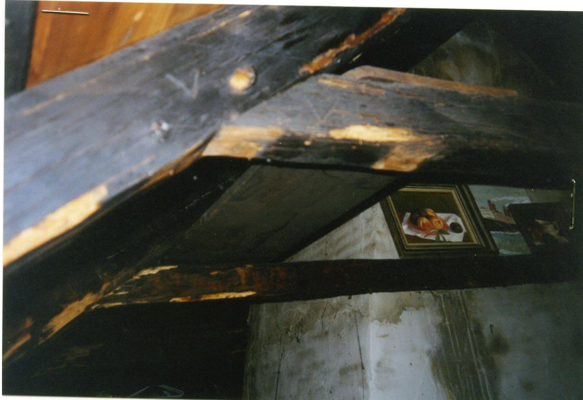
PINNED RAFTER COLLAR, VISIBLE CARPENTER'S MARK
